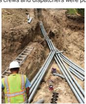
The underground tie line in the Illium Valley (seen here under construction) gives SMPA engineers, operations crews and dispatchers another option to restore power when nature strikes.
